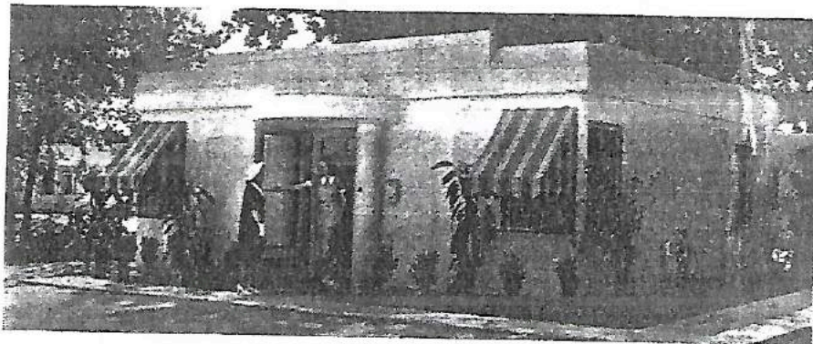
Fig. 1—An arc welded steel 5-room residence of the type which "sailed" across the Illinois River at Peoria, Ill.
